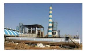
2.9 m Diameter X 56 m Long X 2 Nos Autoclaves.
