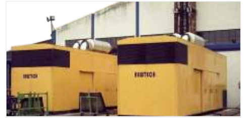
First Acoustic DG Sets 2x1250 KVA installed at Saint Gobain India - 2004
