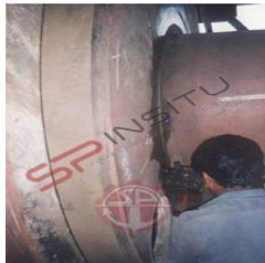
INSITU Machining of seal face location areas in a Cement Industry
