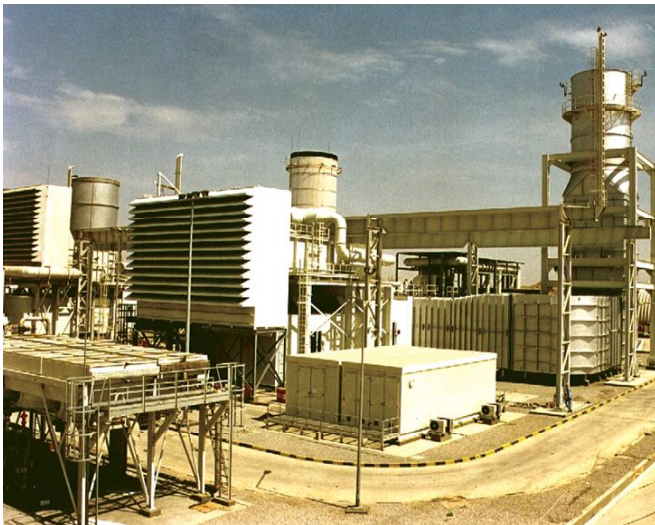
Fr 9E GTG installed at Rusail, Oman
