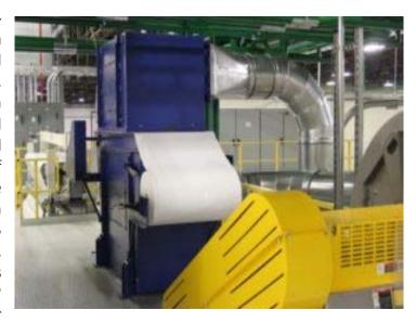
The UHF® system provides for substantially lower space requirements than alternate technologies, resulting in low capital cost. Units come in renewable and non-renewable filter types. Filter replacement is simple and can be performed while the system is on line, for 24/7 operation with no downtime.
