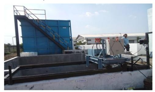
What important news about MBBR system is that its each bio-carrier boosts production level by providing a secured surface area for supporting the growth of heterotrophic and autotrophic bacteria within its cells. It is a high-density population of bacteria, which achieves high-rate biodegradation within the system, while also offering process reliability and ease of operation.
