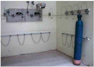
**Gas Cylinder Manifold** is a high pressure structure specially fabricated for interconnecting two or more numbers of cylinders to a common gas supply line when consumption of gas is high. Manifold interconnects two or more number of cylinders for the purpose of availability of more gas at source.
