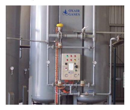
Oxair's oxygen generator can be engineered to integrate with any existing system, or designed from scratch. High purity oxygen is essential for the health and safety of patients and staff alike in medical facilities – the Oxair system delivers constant oxygen of 95.5% purity through PSA filtration.
