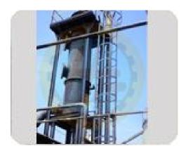
We are one of the well-recognized manufacturers and suppliers of a comprehensive range of Industrial Scrubbers. These are widely used in chemical plants for CL2, SO4, Br and other waste gases. Our offered range is fabricated by our professionals using high grade FRP, PP/FRP, PVC/FRP. These are designed and developed with high precision in order to meet the international quality standards. We offer these scrubbers in various specifications to fulfill the wide needs of the clients.
