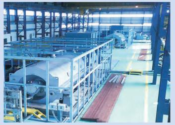
Acoustic Enclosure Installed around the turbo blower
