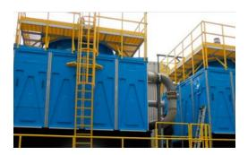
BCS is one of the leading manufacturers of compact and space saving FRP cooling towers. In FRP cooling towers, multiple fibers are joined mutually and are available in form of mat. The mat is joined together with polyester resin, accelerator and catalyst. We deal with both Round Shaped and Square shaped towers
