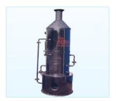
The construction is of a packaged type vertical design multistage shell and tube boiler. The water is in the shell side and the flue gases of combustion travel through the tubes in the shell. This is a rugged design boiler which can withstand a higher degree of hardness in the water. Blowdown valves are provided for removal of TDS in the boiler water.
