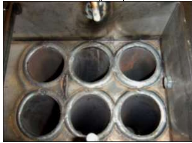
The tubes shown on this picture without the flue gas break that you can see on the picture to the left.
