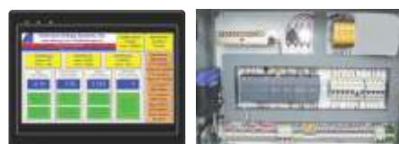
Typical Touch Screen Operator Interface. Siemens S7-1200 PLC with Ethernet Interface and DSLRouter.
