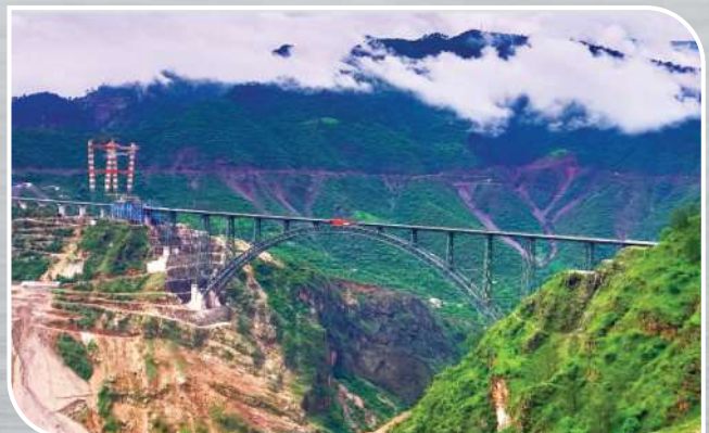
Chenab Rail Bridge, Jammu & Kashmir
